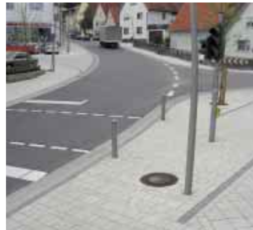
Invisible VS 5 technology: partial view of the finished work.
