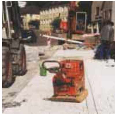
First construction phase: paving work with VS 5.
