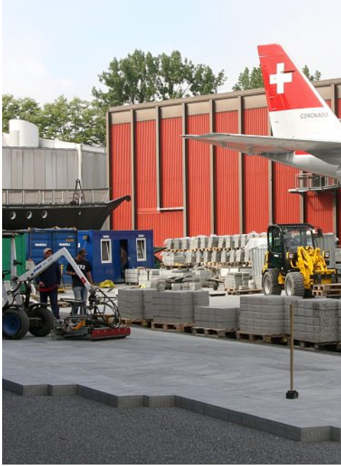
Mechanized laying of VS 5 pavers in June 2009; paver depth: 12.8 cm
