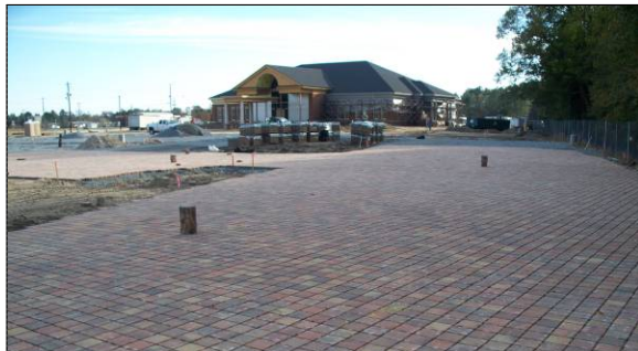
Parking lot under construction
