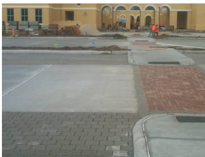
Installing SF-Rima® permeable pavement
