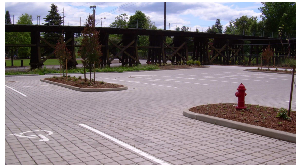
SF-Rima™ parking lot and rain garden in background
