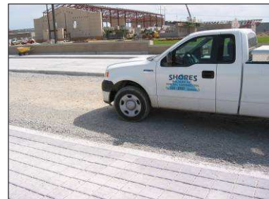
The travel lanes will be paved with concrete.
