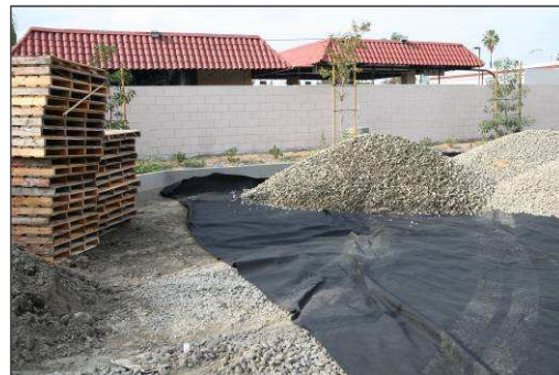
Storage of material used for this SF-Rima™ pavement.
